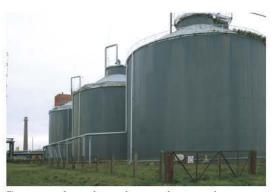
Figure 10.14. Anaerobic methane production tanks at a wastewater treatment plant (Rīga, Latvia)
