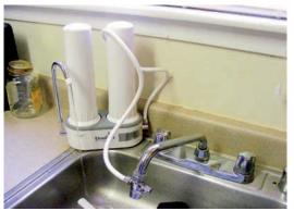
Figure 10.13. Personal water treatment device that can be connected to the tap
